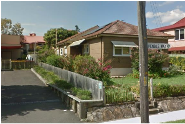
Pendle Way (edge of site, west of the Village)*
